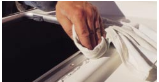
Clean up the excess bedding compound
