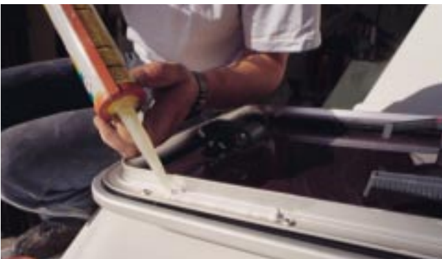
Apply sealant to both sides of fasten holes on the hatch frame. If replacing an existing hatch fill any old fixing holes with sealant.
