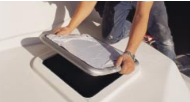
Test fit the hatch before applying sealant.
